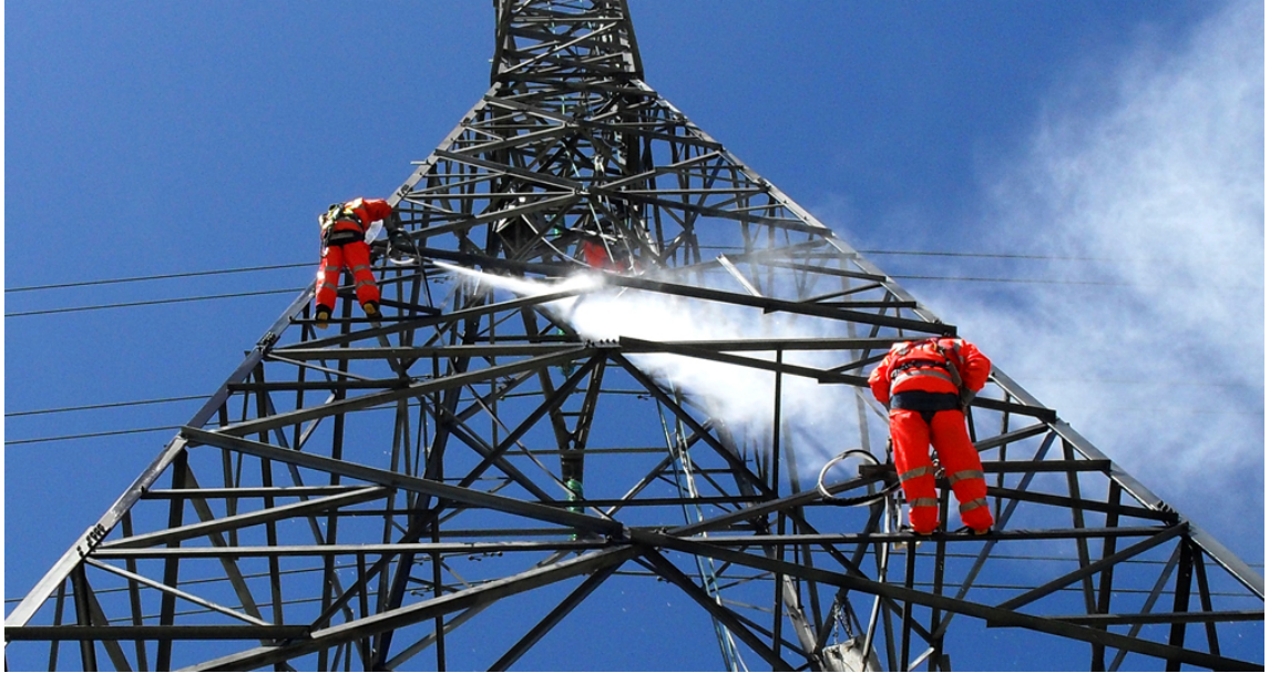
FIGURE 1.1: Workers performing maintenance of a power transmission tower [11]
