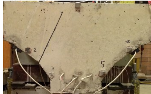
Figure 5. Damage case 3, (225 × 50) mm cut in the concrete
