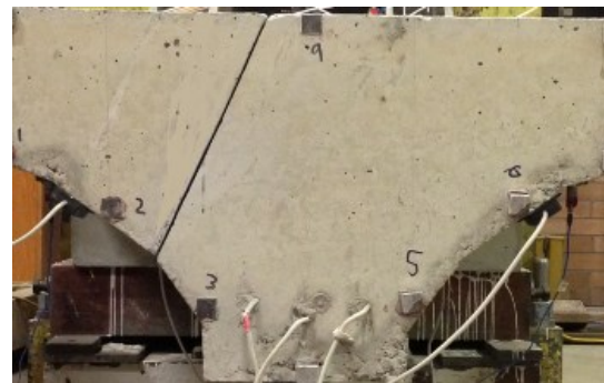
Figure 6. Damage case 4, (270 × 50) mm cut in the concrete
