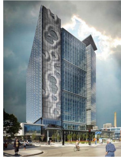
Figure 7 - Rendering of non-repetitive bespoke high rise building cladding (courtesy of Laing O'Rourke)
