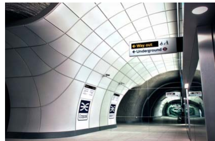
Figure 1 - Photo of Crossrail tunnel intersection mockup (courtesy of Laing O'Rourke)
