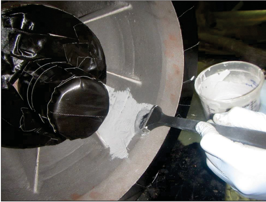
Figure 90 – Coating being applied to surface
