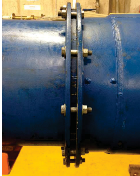
Figure 231 – Assembled dismantling joint
