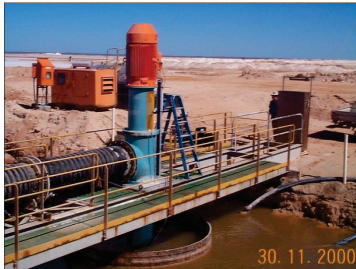
Figure 5 – 450AX 'Ornel' pump, for water transfer (Installation by Weir Minerals Australia)
