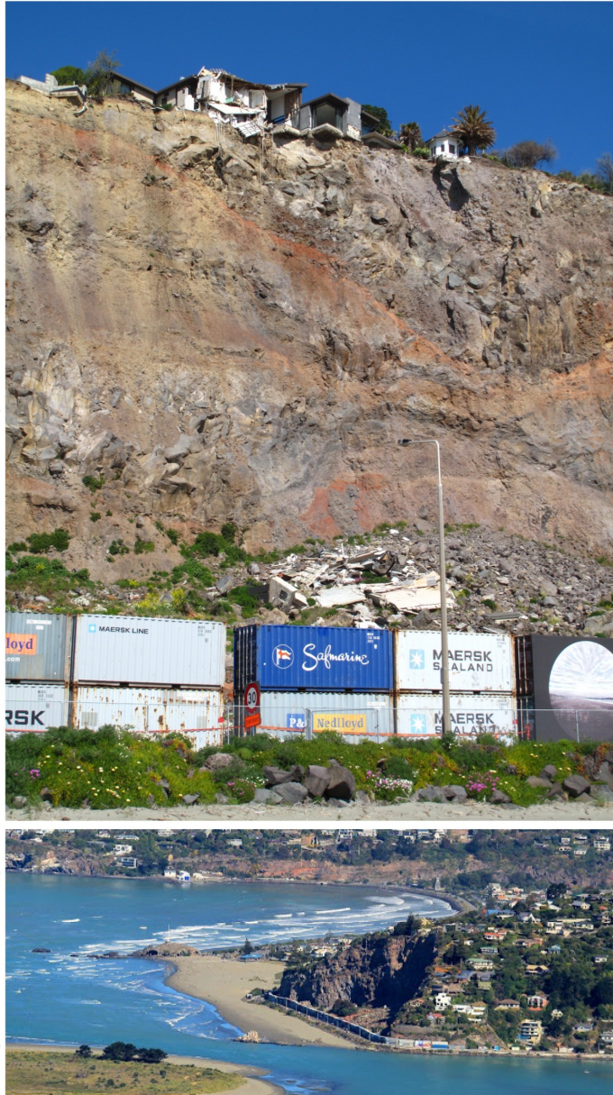
Figure 2. The collapse of Christchurch's Port Hills in the 2010/11, where fallen cliff faces have not only led to loss of property, but have also threatened access and recreation opportunities. There is now tension between community and government on the rebuilding of the road, pathways and other open space facilities (sources top: N. Jones; below: BeckerFraser Photos).
