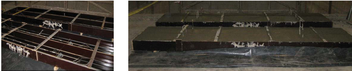
Figure 7.1: Slab moulds before and after pouring of lightweight concrete
