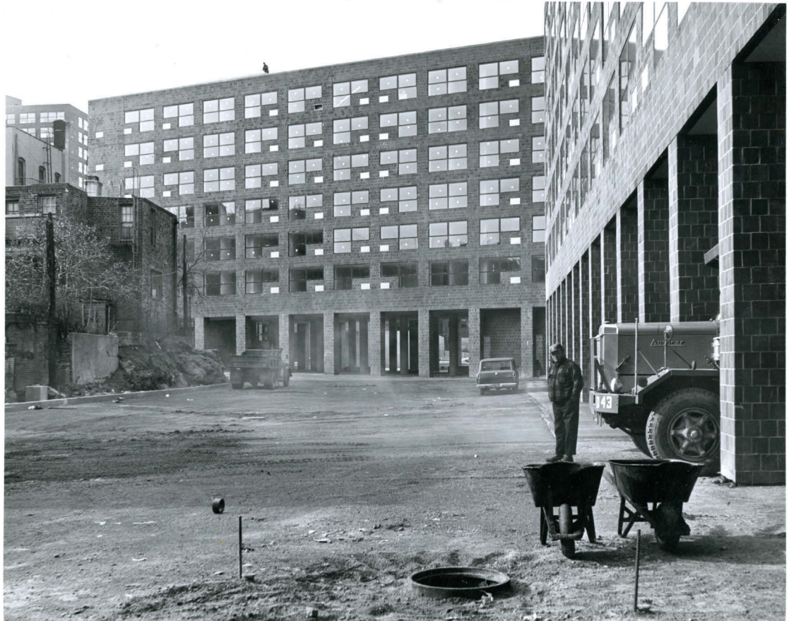
Image 17: Twin Parks Northeast. Under construction. Source: Courtesy Richard Meier & Partners Architects
