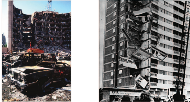
Figure 1. Structural progressive collapse induced by blast loads Left: 1995 Alfred P. Murrah Federal Building ( http://en.wikipedia.org/wiki/Alfred_P._Murrah_Federal_Building ) Right: 1968 Ronan Point Building ( http://en.wikipedia.org/wiki/Ronan_Point )
