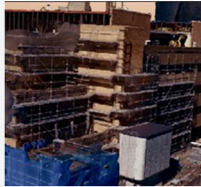
Figure 2: Building exterior data captured by drone.
