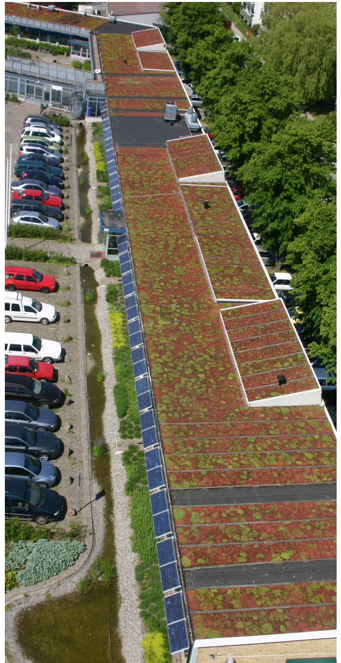
Augustenborg Botanical Roof Garden, Malmö (source: L. Lundberg, n.d.)
