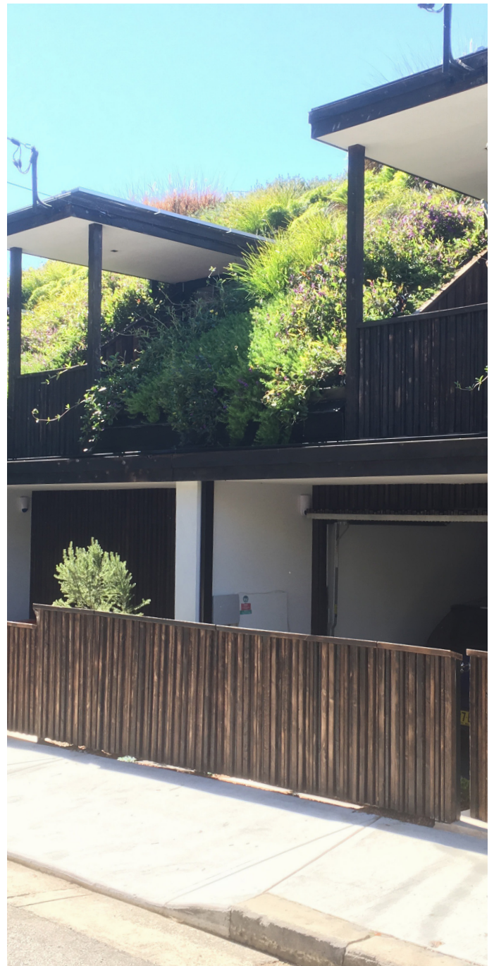
A green roof on a pitched roof in Newtown, Sydney (source: S.Wilkinson, 2016)
