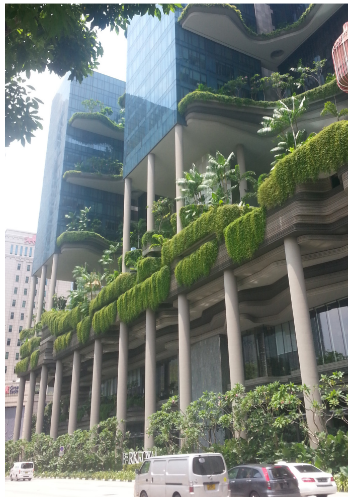
The Parkroyal on Pickering in Singapore features a range of vertical greening (source: N.Pelleri, 2017)
