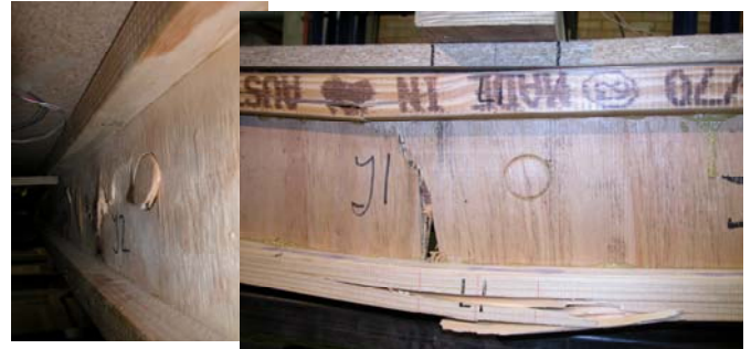
Figure 7: shear failure of I-joist web (left) & tensile failure of I-joist flange (right)
