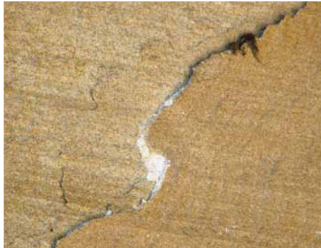
Figure 2.3. Photo illustrating subflorescence as a result of accumulated salts below the sandstone surface (Swann 2011)
