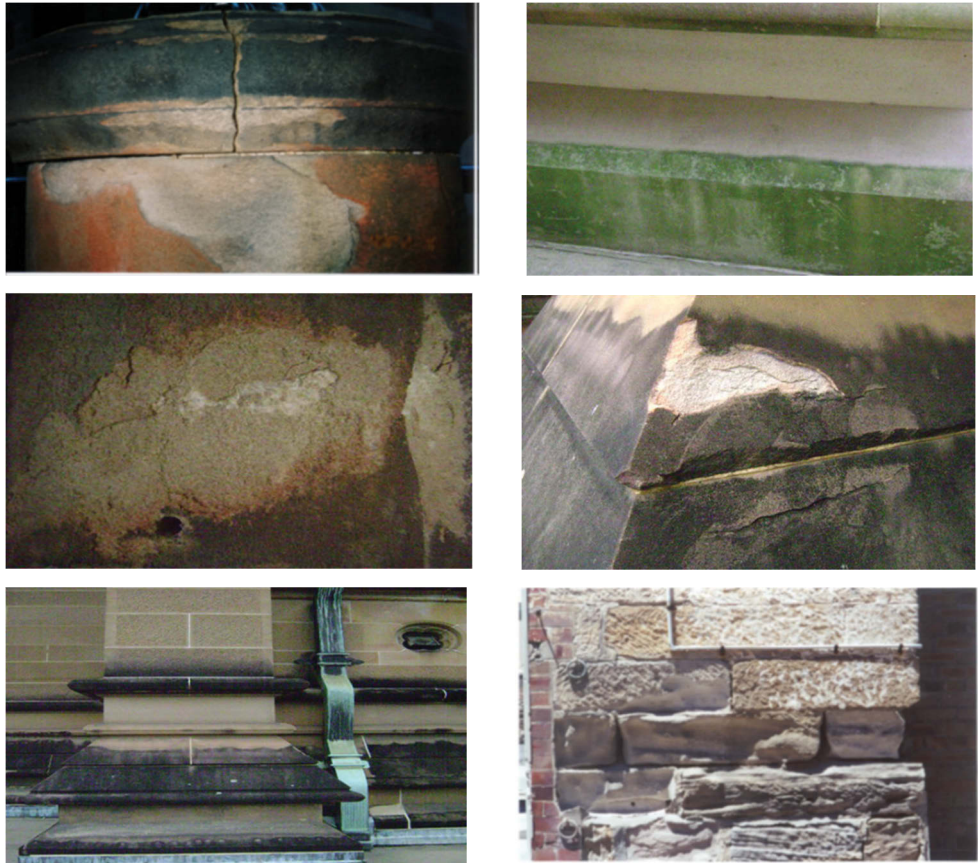
Figure 2.5. Deterioration of heritage sandstones taken from St Mary Cathedral in Sydney showing cracking, discoloration, detachment, biological colonization and granular disintegration (Ip 2007)
