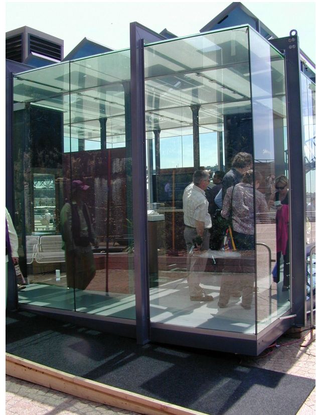
Fig. 4. The ‘NanoHouse’, a glass structure designed to demonstrate the best of radiative and convective heat transfer control in a structure exposed to subtropical sunlight (photo, MB Cortie).
