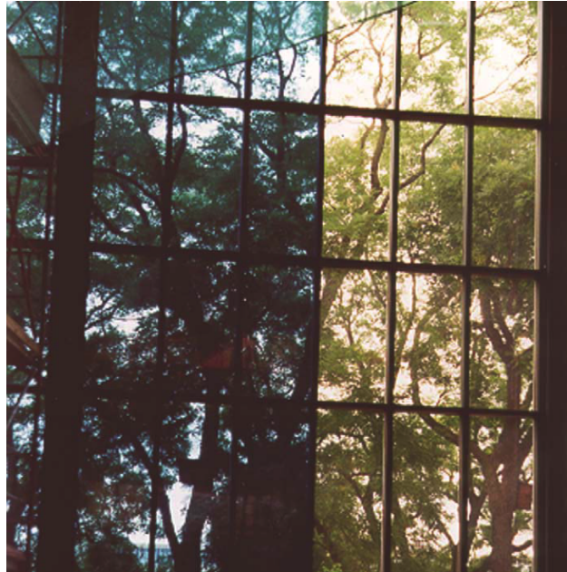
Fig. 10. An electrochromic window with the left side switched to near-IR and glare blocking mode, and the right side clear. This window was produced by Flabeg and reported by Lampert [47]. Permitted under creative commons license, http://creativecommons.org/licenses/by-nc-nd/3.0/
