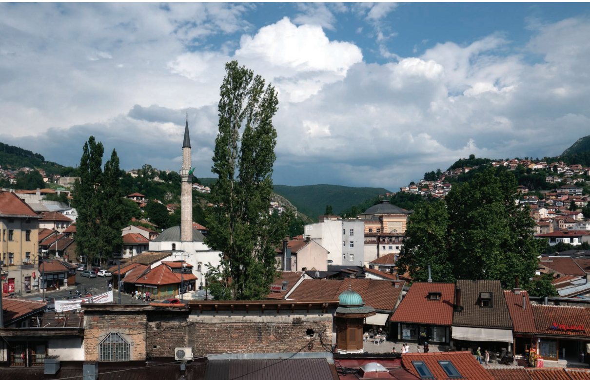
Fig. 04: The Baščaršija and its Ottoman influenced architecture, and the pseudo-Moorish Vijećnica in the background.
