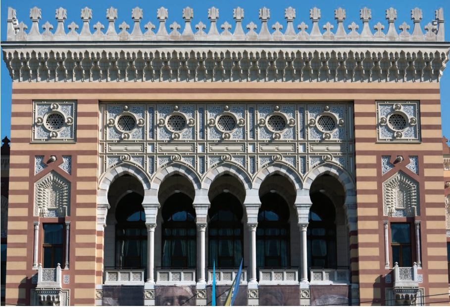
Fig. 06: Architectonic details on the front façade of the Vijećnica.
