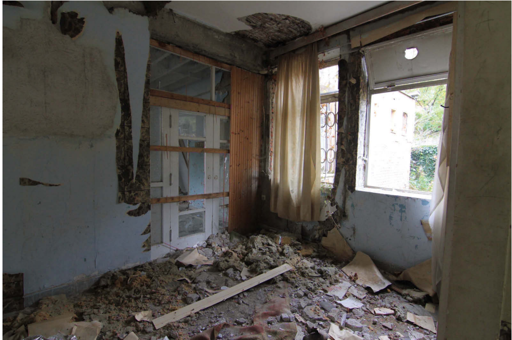
Figure 124: Interior of Banjska sanatorium (Nevena Mrdjenovic 2013)
