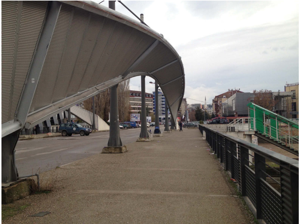
Figure 139: Mitrovica Bridge from the North (Nevena Mrdjenovic 2013)
