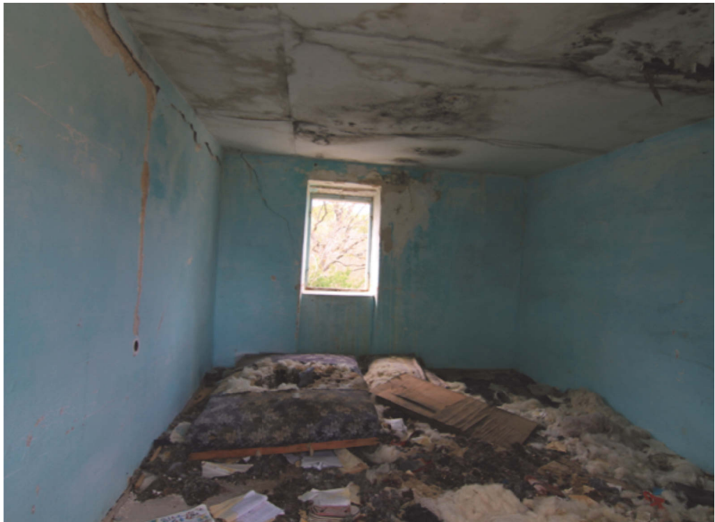
Figure 72: Demolished bedroom (Nevena Mrdjenovic 2014)
