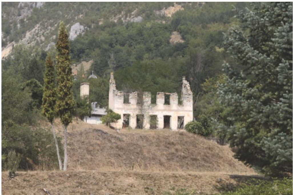
Figure 80: Destroyed dwelling in a village near Visegrad (Nevena Mrdjenovic 2012)
