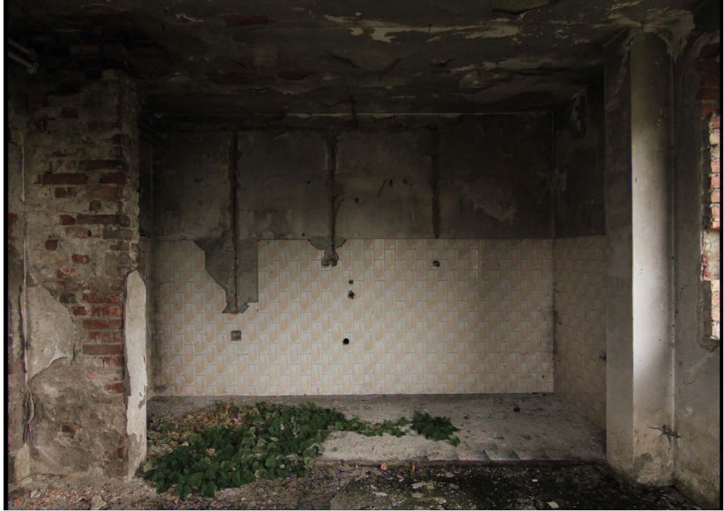
Figure 106: A former kitchen (Nevena Mrdjenovic 2013)
