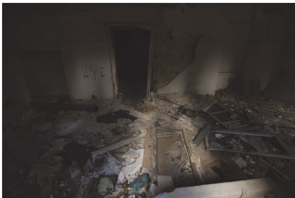
Figure 60: The basement viewed from a courtyard window (Nevena Mrdjenovic 2011)
