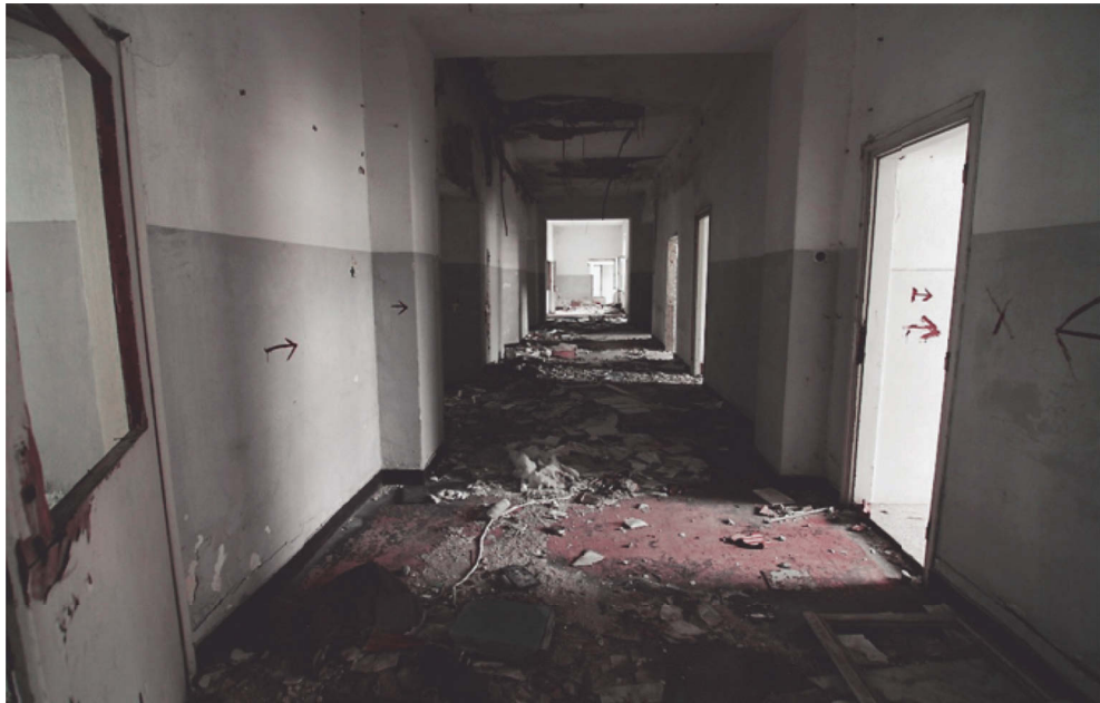
Figure 51: Hallways of abandoned hospital in Knin (Nevena Mrdjenovic 2011)
