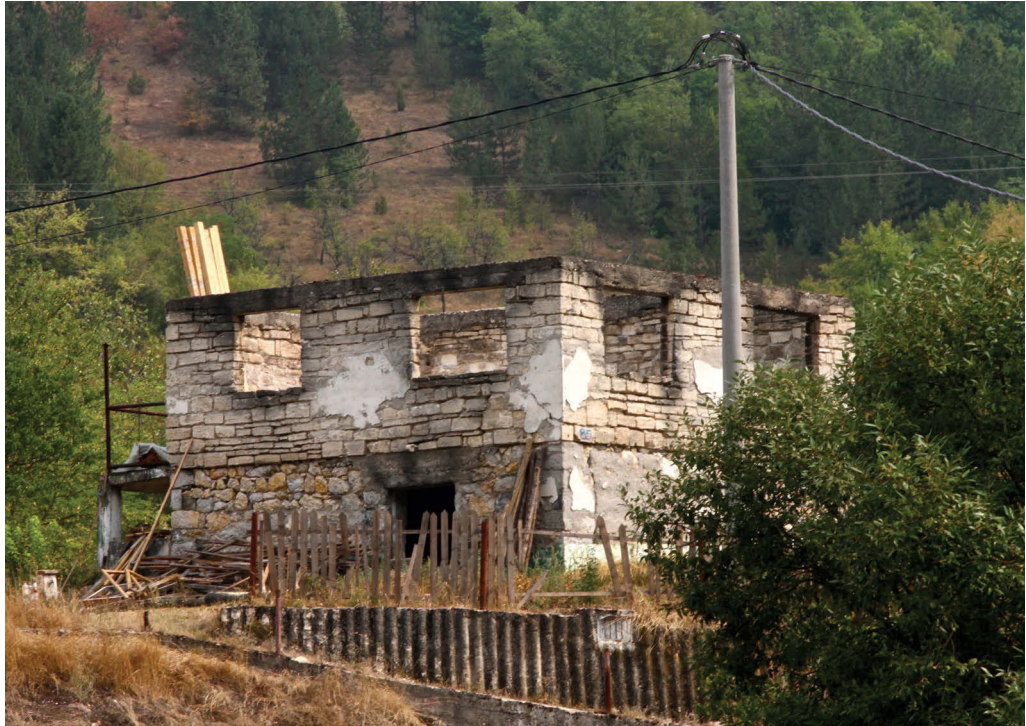
Figure 85: War-torn house in a village near Visegrad (Nevena Mrdjenovic 2012)
