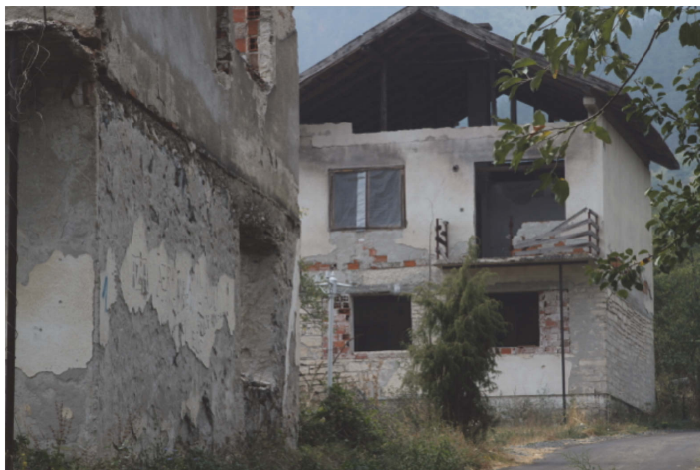
Figure 84: An abandoned house in Visegrad (Nevena Mrdjenovic 2012)
