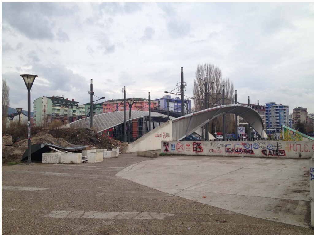
Figure 138: Mitrovica Bridge (Nevena Mrdjenovic 2013)
