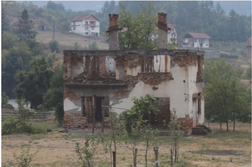
Figure 79: War-torn and abandoned houses near Visegrad (Nevena Mrdjenovic 2012)
