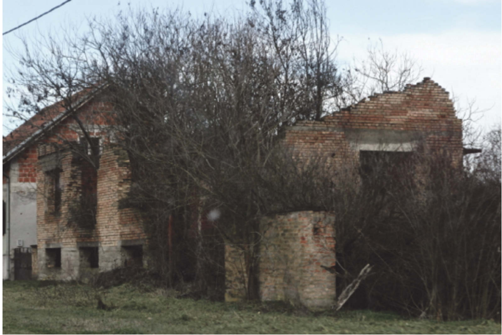
Figure 94: Demolished houses on E-661 (Nevena Mrdjenovic 2012)
