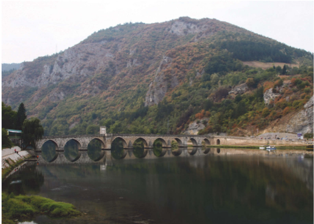
Figure 82: Mehmed Pasa Sokolovic Bridge Visegrad (Nevena Mrdjenovic 2012)
