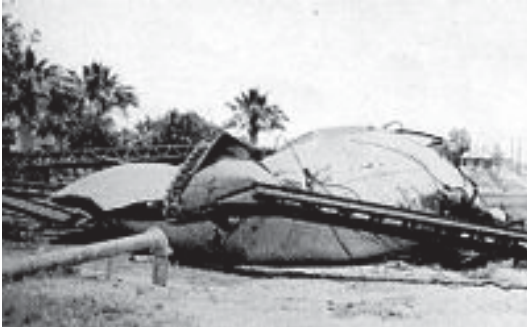
(c) Imperial's 100,000 gallon water tank that collapsed in the earthquake (Photo: U.S. Coast and Geodetic Survey, Hemple 1941)
