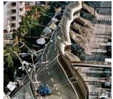
(e) 1 km of Hanshin expressway collapsed (from JMA library, Koketsu et al. 1998)
