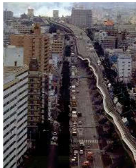
(e) 1 km of Hanshin expressway collapsed (from JMA library, Koketsu et al. 1998)
