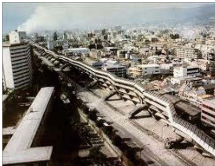
(e) 1 km of Hanshin expressway collapsed (from JMA library, Koketsu et al. 1998)
