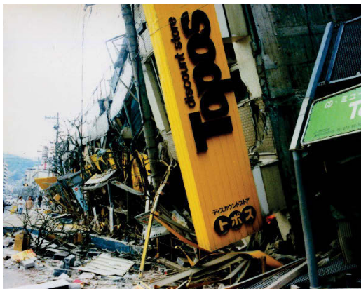
c) Damage at Minatogawa, Kobe (from JMA library, Koketsu et al. 1998)
