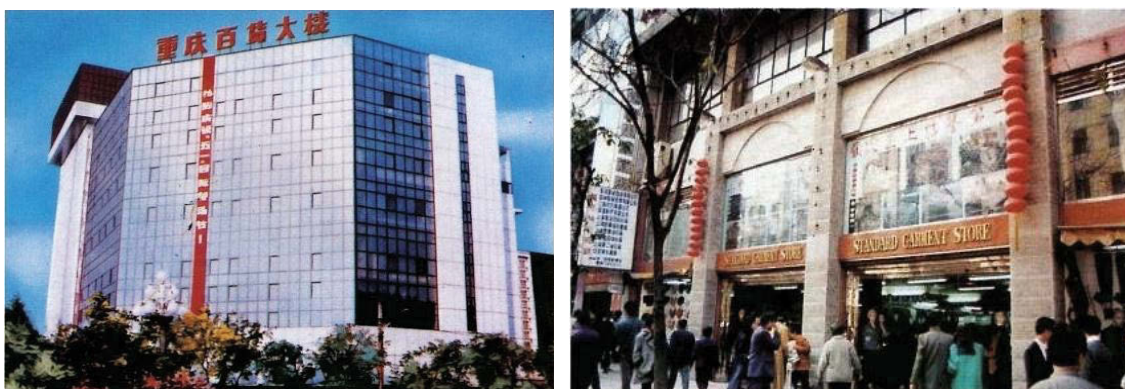
Fig 3.8 Chongqing Jiefangbei department store, a typical commercial space in the 1980s
