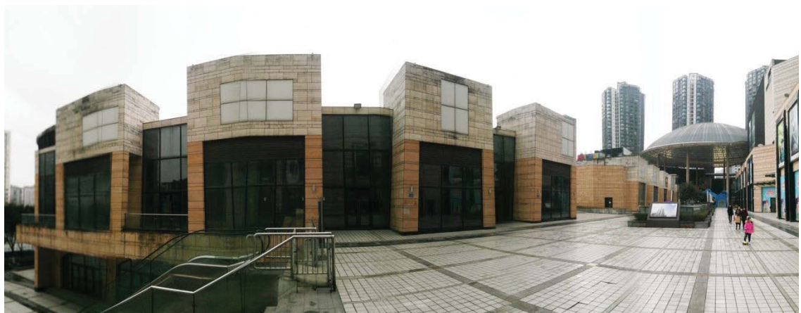
Fig 5.1 A large scale commercial complex in the central urban area of Chongqing (The shopping spaces of this complex have never been fully used. Those shops in the photo have been empty since 2008 when the complex was opened to the public).
