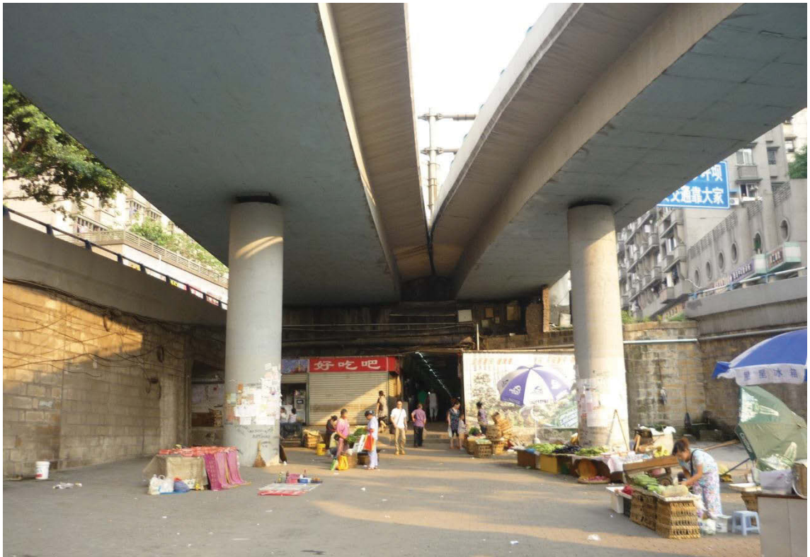
Fig 4.6 Urban space under an elevated highway utilised as a fruit market in Chongqing
