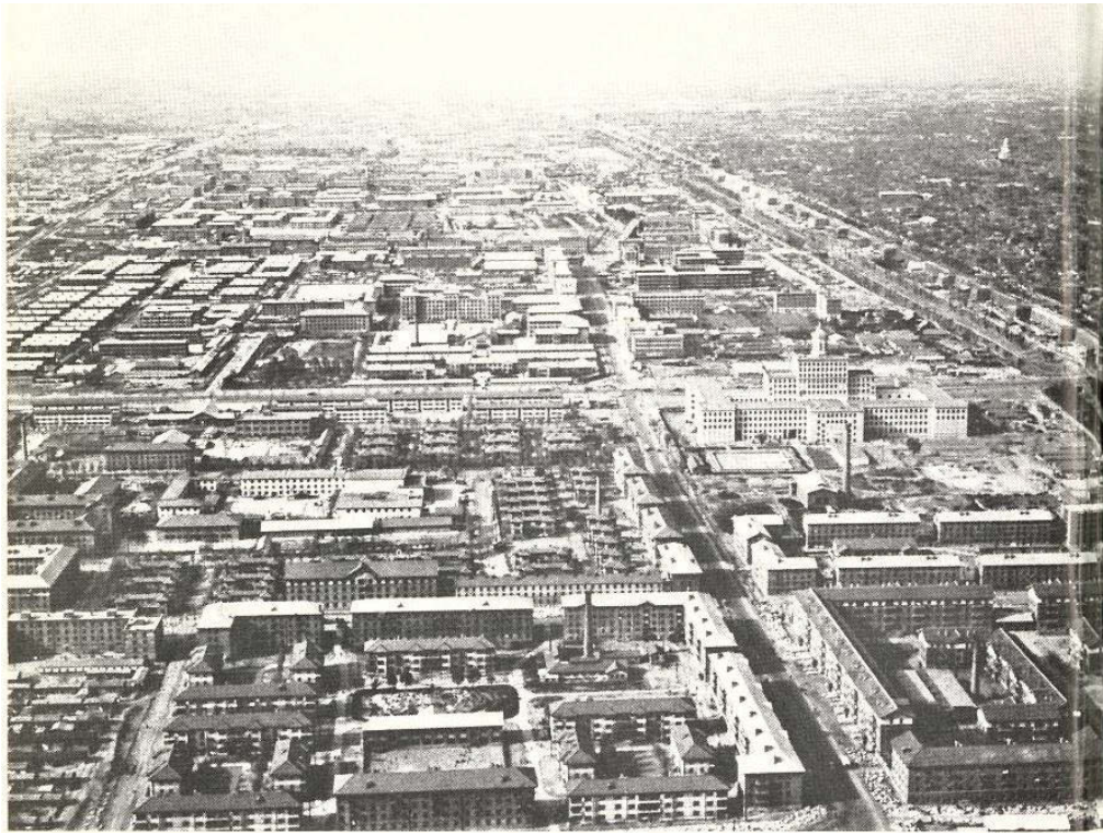
Fig 3.2 The suburb of Beijing in Mao's era (As a 'production centre', the space was structured by a series of 'self-sufficient' work-units based on the Soviet mikrorayon model)
