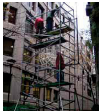
Figure 4.26 Installing the Web of Light
