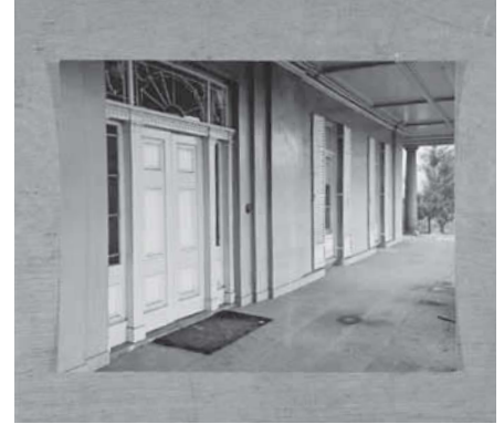
Figure 4.27 Example of transom windows and side lights in an historic building (Stacey 1968, p.27)
