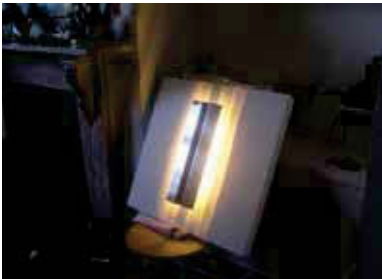
Figure 5.30 Reflection Lightlouvre in Household 4 in vestibule area.
