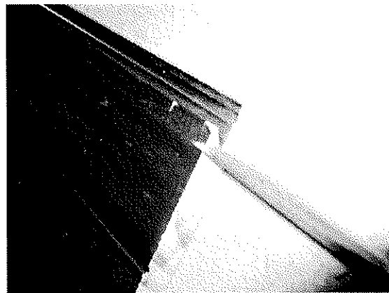
Figure 9: Connector (with adhesive applied) fitted behind board
