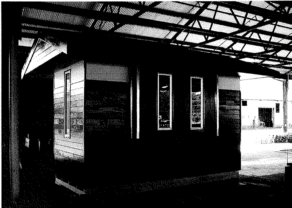
Figure 2: The Flatline prototype building
