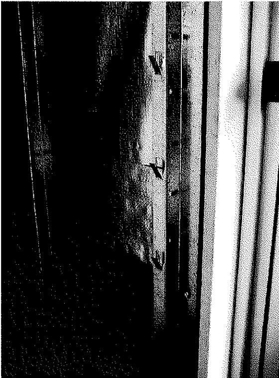
Figure 5: Metal battens fixed to the face of studs with fins protruding
