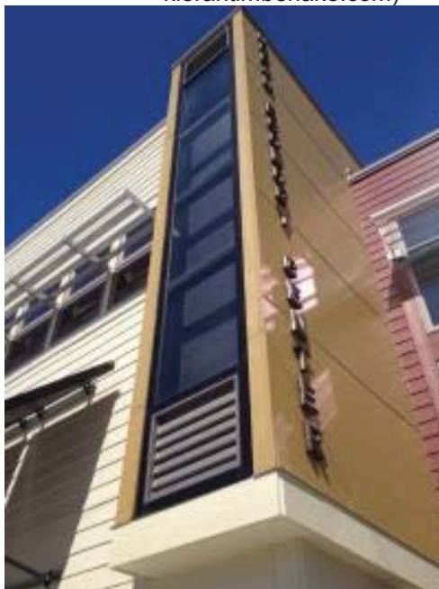
Figure 1.18. Solar Chimneys installed at the roof of Sidwell Friends School, Washington DC. (Source: By Peter Aaron/OTTO, taken from kierantimberlake.com )
