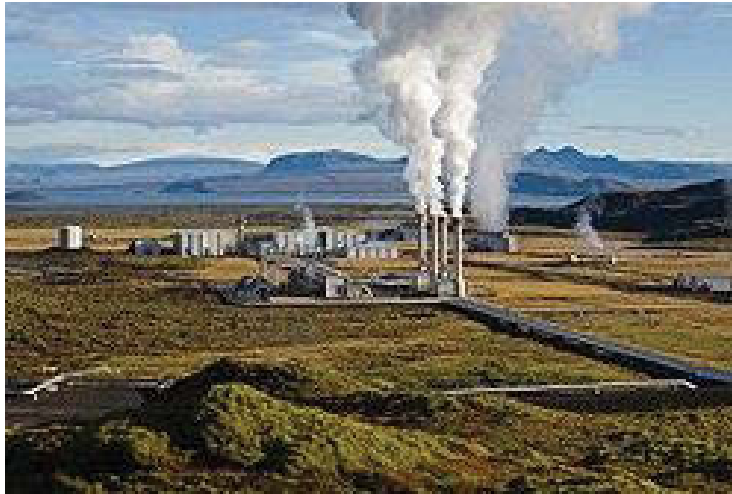
Figure:1.10: Example of Geo Thermal Energy Plant - Nesjavellir Geothermal Power Station in Iceland (Source: Photo by Gretar Ívarsson, geologist at Nesjavellir (Public Domain), taken from Wikipedia)
