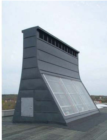
Figure:1.14a: An example of Solar Chimney Installed at a Building for Natural Ventilation - Tanga School Falkenberg, Sweden (Source: Photo Taken from “new-learn.info”)
