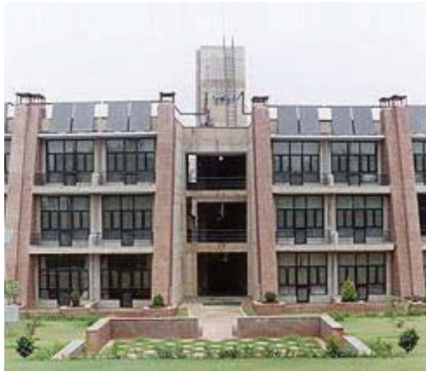
Figure 1.16 Chimneys built for natural ventilation at The Energy and Resources Institute (TERI), Delhi, India. (Source: “ teriin.org/technology/energy-efficient ”)
