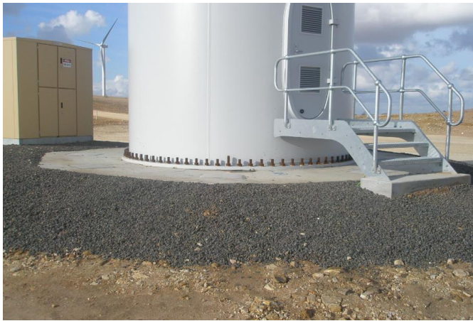
Fig. 11. An example of gravel installation around turbine tower base
