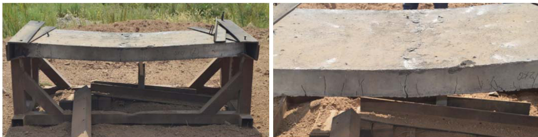
Fig. 7: SWM-3 slab after 12 kg TNT detonation from 1.5 m standoff distance
