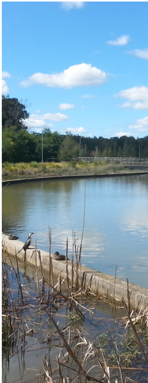
Constructed wetlands along Caddies Creek, Rouse Hill manage and treat urban stormwater, provide recreation opportunities and create urban habitat
