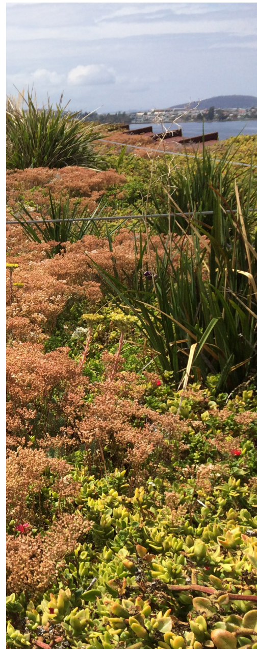
The green roof at MONA, Hobart contributes to urban greening in Hobart
