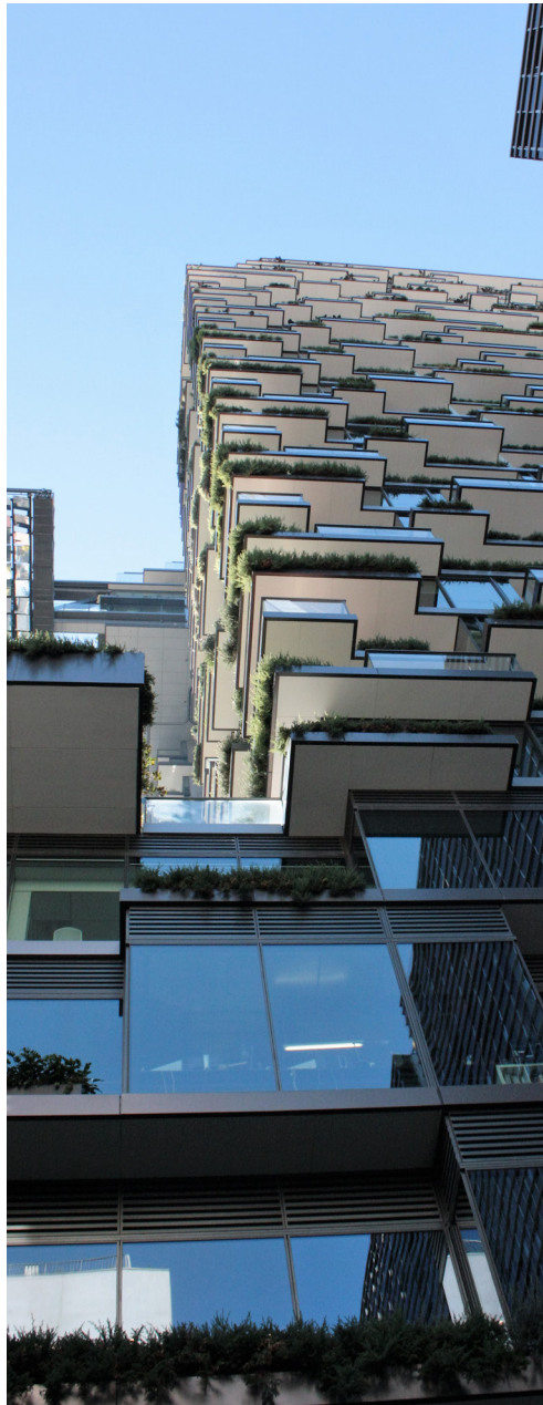
Vertical greening is integrated into the balcony design at One Central Park, Chippendale
