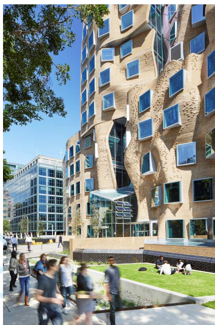
Image 1. Dr Chau Chak Wing Building, Sydney, Australia
