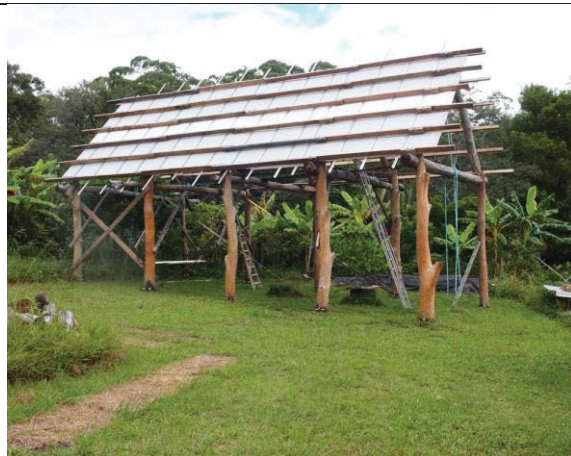
j) Bush carpentry house under construction
