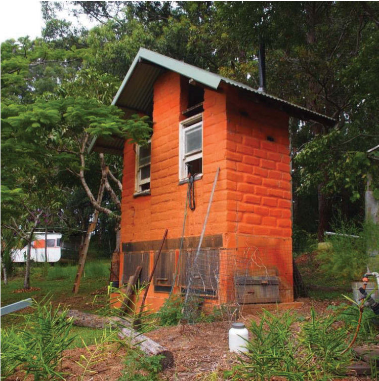
Figure 6-7: Mudbrick composting toilet 'block', with toilets. Note the raised level of the building to allow the composting chambers, which can be accessed from the hatches on the side.
