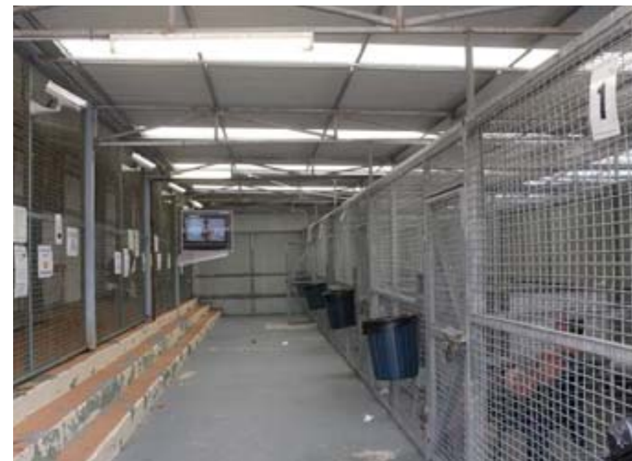
Long Bay holding yard
