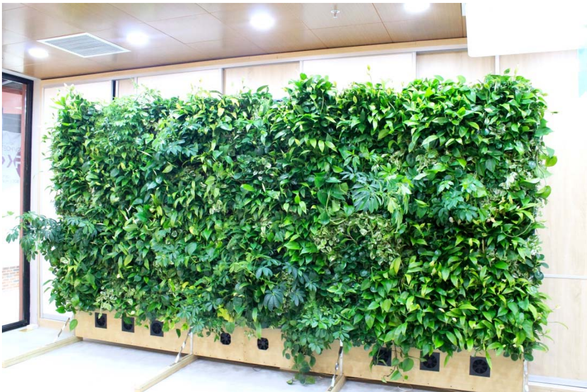
Figure 3. The active green wall used to filter ambient PM and VOCs installed in a classroom in Beijing, China.
