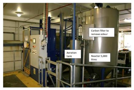
The technology used by Active Research at Federation Square and similar AD systems is a high rate fixed film anaerobic digestion, enhanced reactor technology including constant mix, insulated reactors, scum removal, heating, retentive thickening and remote management capability through the utilisation of best practise electronic monitoring equipment. A typical process schematic is shown below (Active Research).
