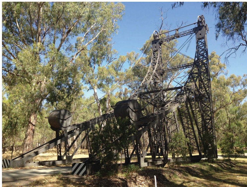
FIGURE 6.6. Old bridge at Darlington Point, NSW, 2015 Image courtesy Jonathan Jones
