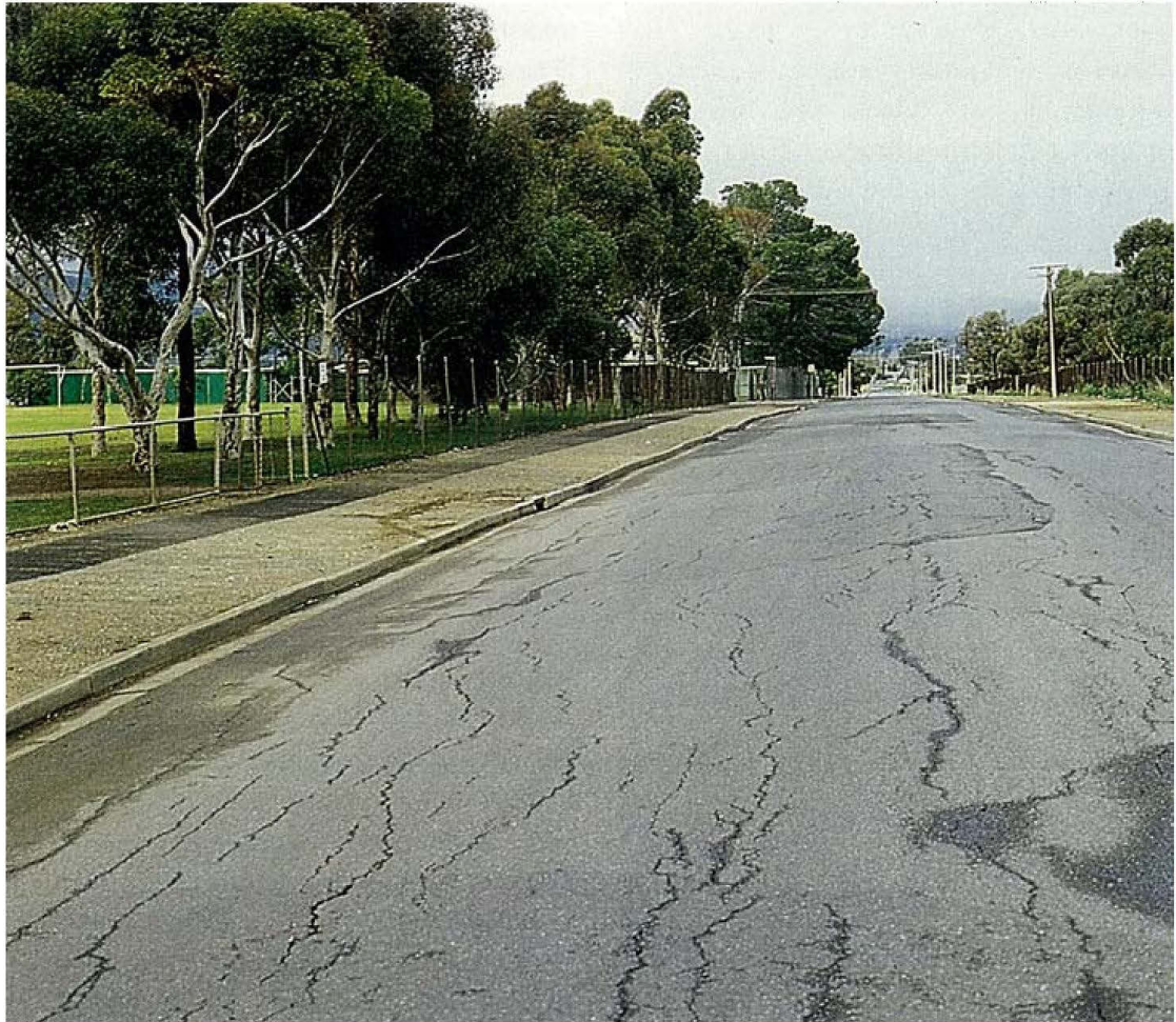
Figure 1.2 A cracked road in Adelaide, Australia after (Considine 1984)
