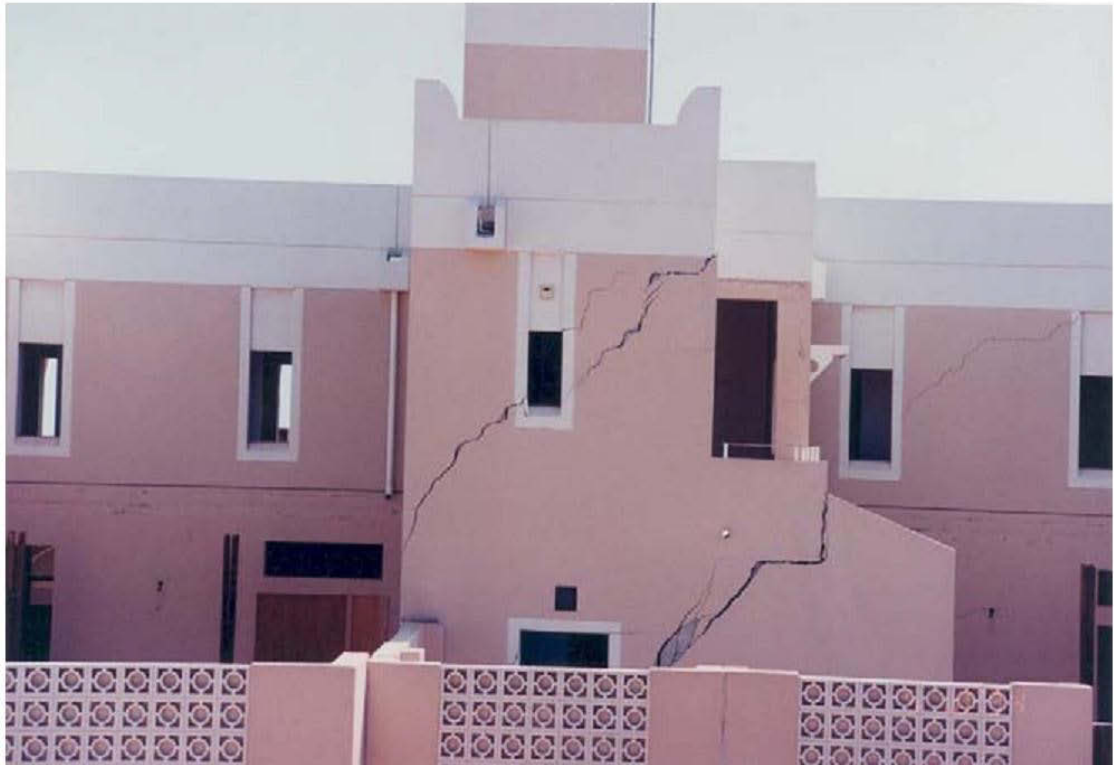
Figure 1.1 Structural damage due to ground heaving after (Al-Rawas et al. 2005)
