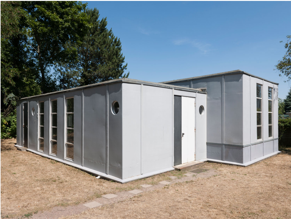
Figure 7. Steel House (Richard Paulick and Georg Muche 1926-27). Photo: Thomas Meyer, Ostkreuz 2018.
