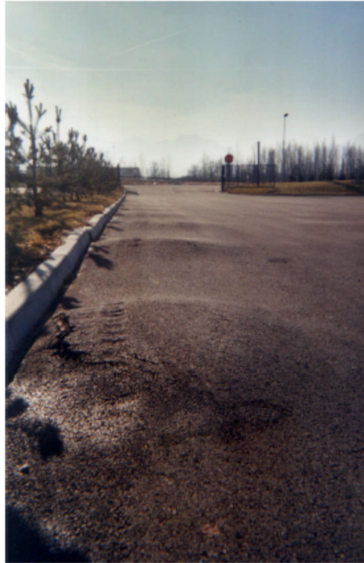
Figure 2.13 Egg carton (or mushroom) effect on rigid inclusions (ASIRI 2012)
