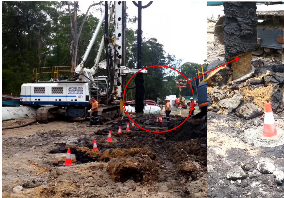
Figure 1.1 CIC installation, Heathcote project, NSW, Australia
