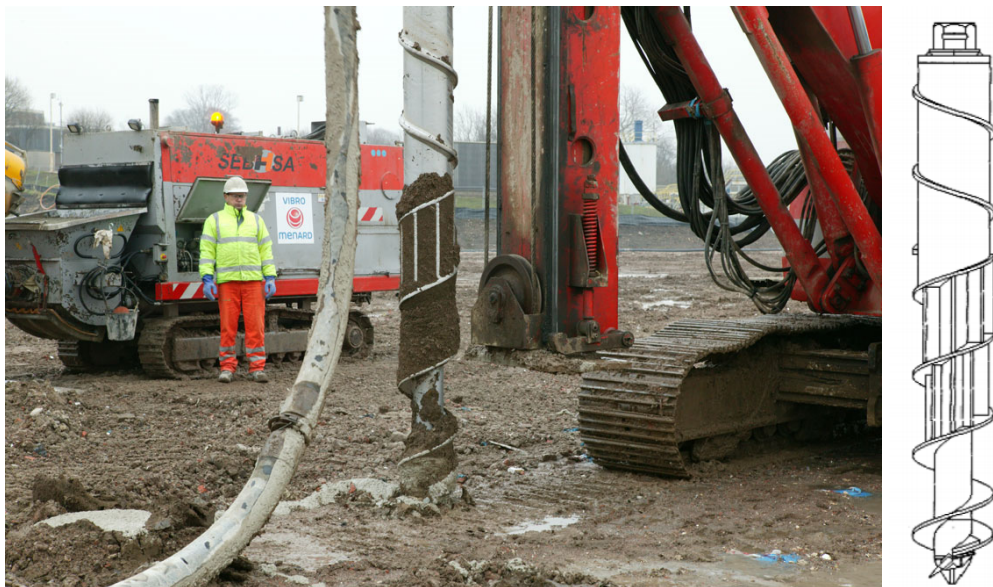
Figure 2.2 CIC Installation augers (Courtesy of Menard 2018).
