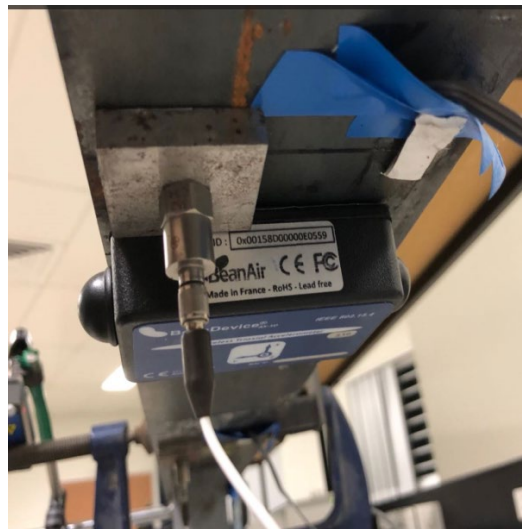
(c) Wireless sensor on the bridge
