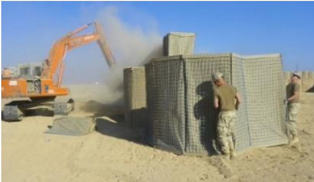
Figure 12: Building Delaram FOB [77]
