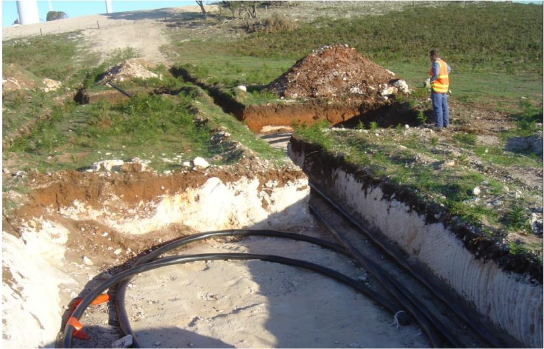
Figure 4-17: Three core 33 kV cable joint bay (courtesy of Aurecon).
