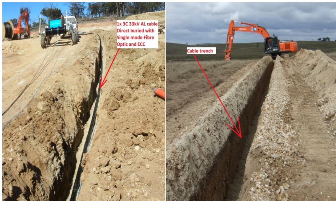
Figure 2-10: Cable installation for wind farm (courtesy of Aurecon)
