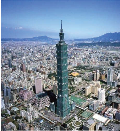
Figure 2.10 Taipei 101 building by CTBUH.
