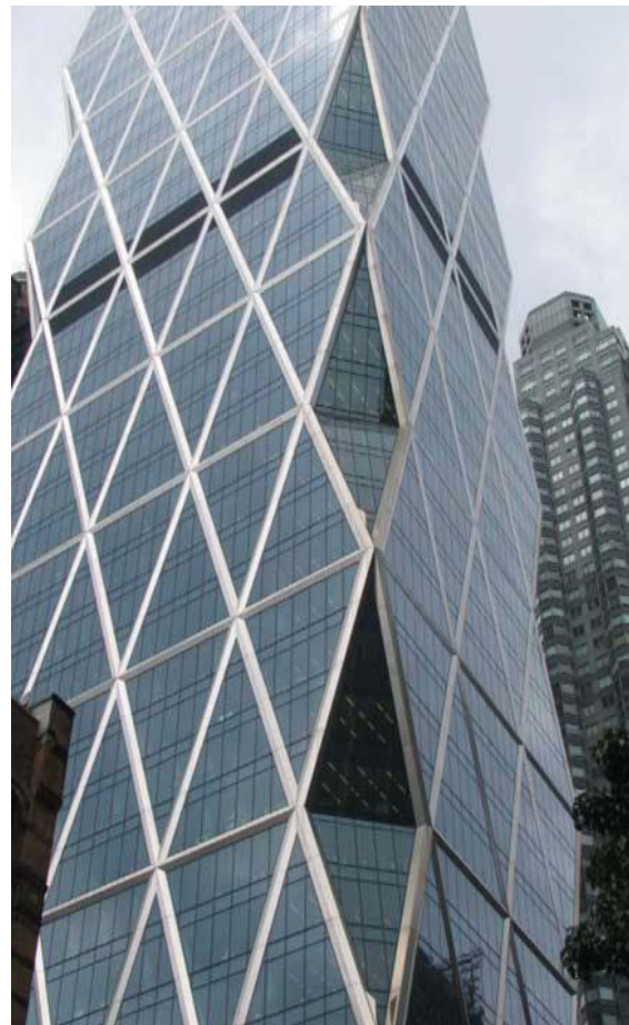
Figure 2.7 Chamfered Corner by CTBUH.
