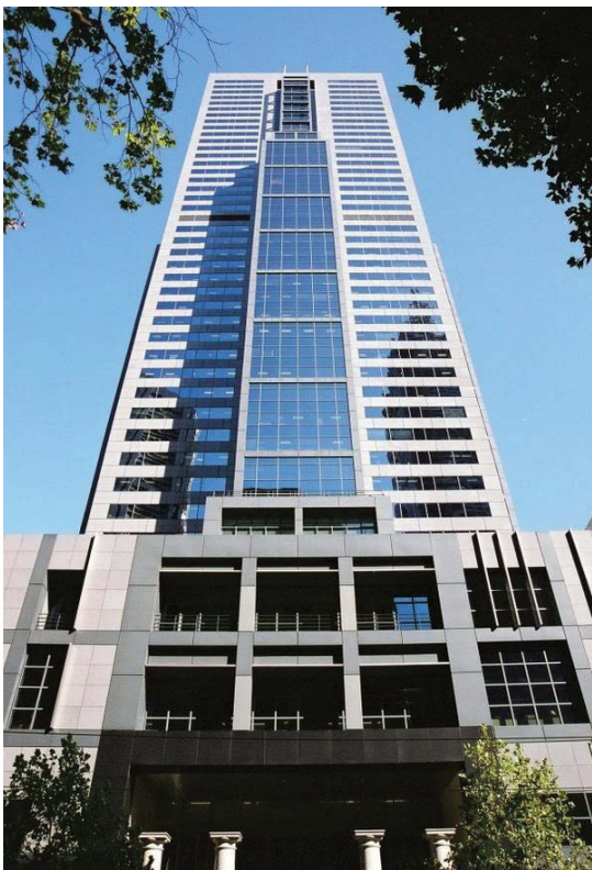
Figure 6.1b Existing Tall Building Design by CTBUH
