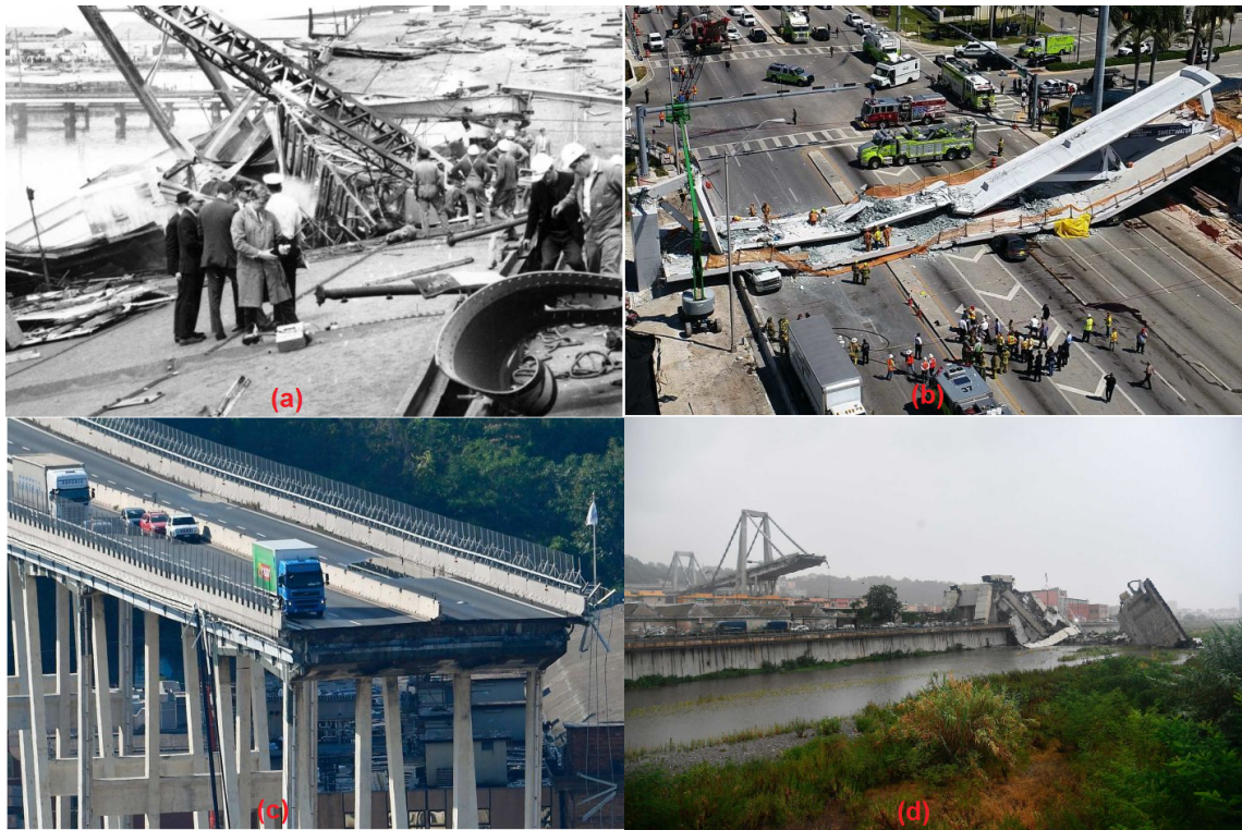
Figure 1.3 : Worldwide bridges collapse, a sign of things to come if infrastructure maintenance is ignored,
