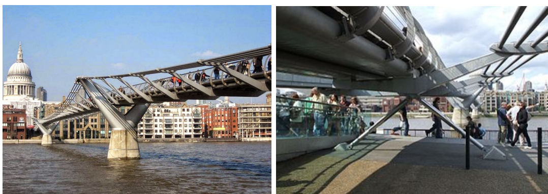
(a) The Millennium bridge.
