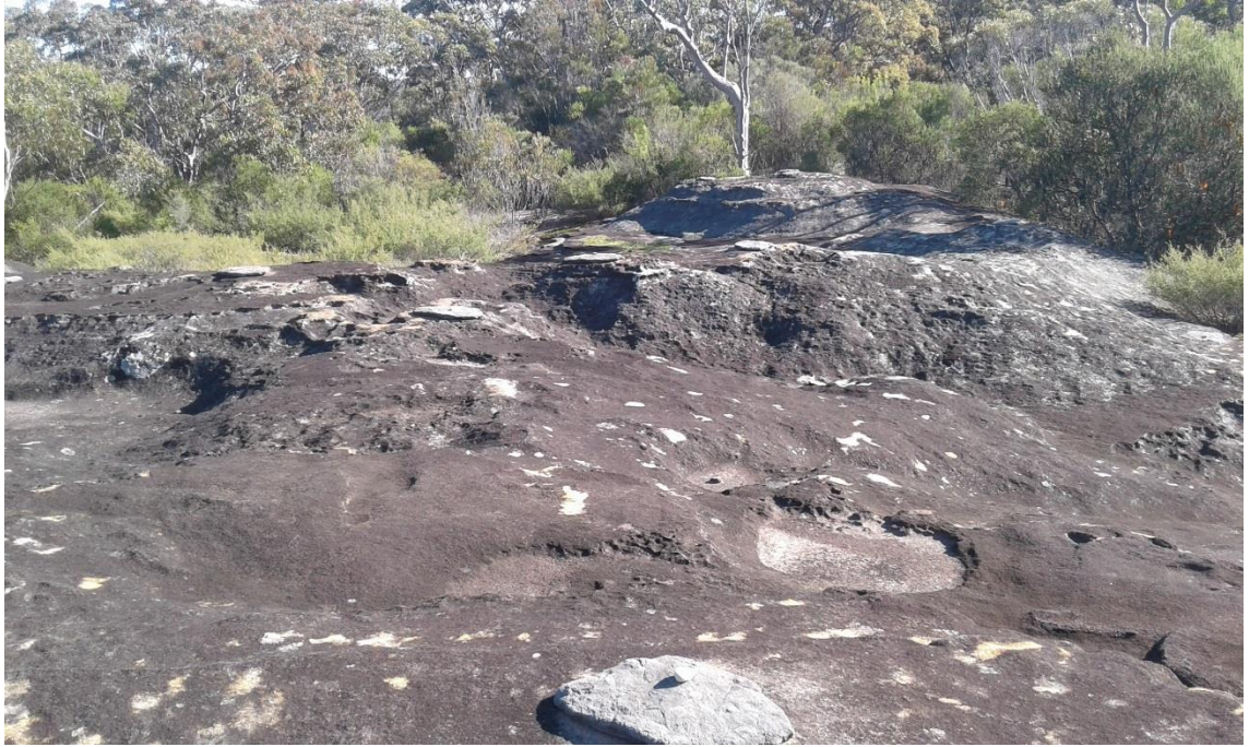
Figure 2-2 Restored artificial rocks made up of fibre reinforced concrete in Dharawal national park.
