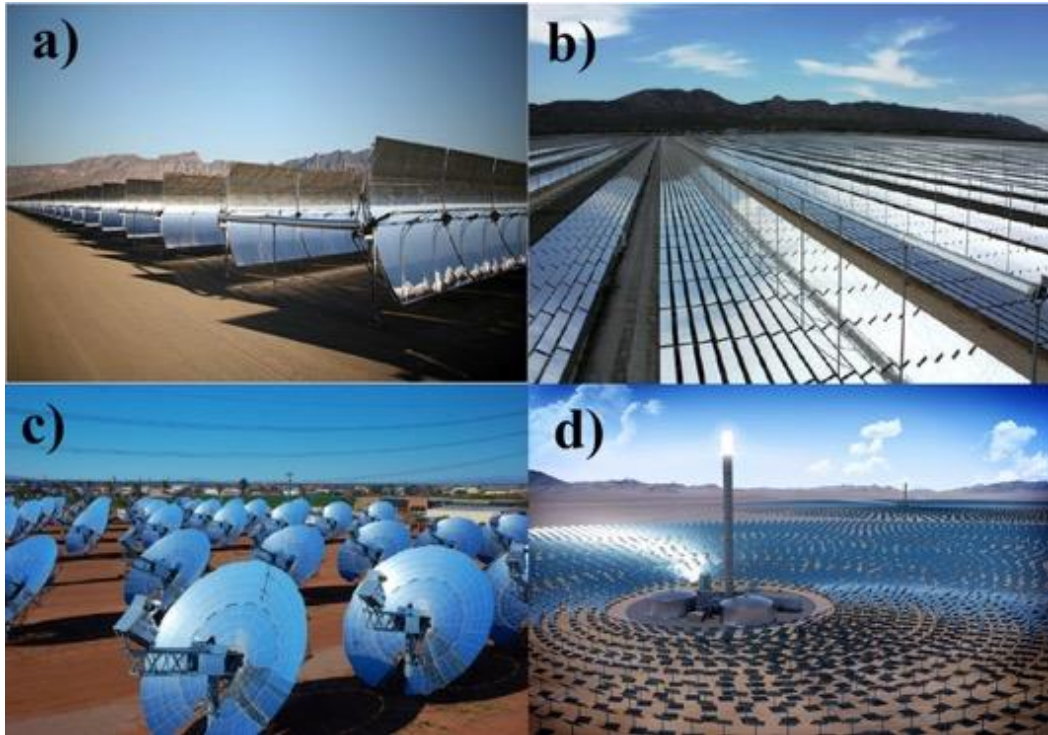
Figure 1.4 – Types of concentrated solar power plants. a) Parabolic trough b) Linear Fresnel reflector c) Parabolic dish d) Solar power tower, photos are from reference [3] with the permission under the terms of the Creative Commons Attribution 3.0 License
