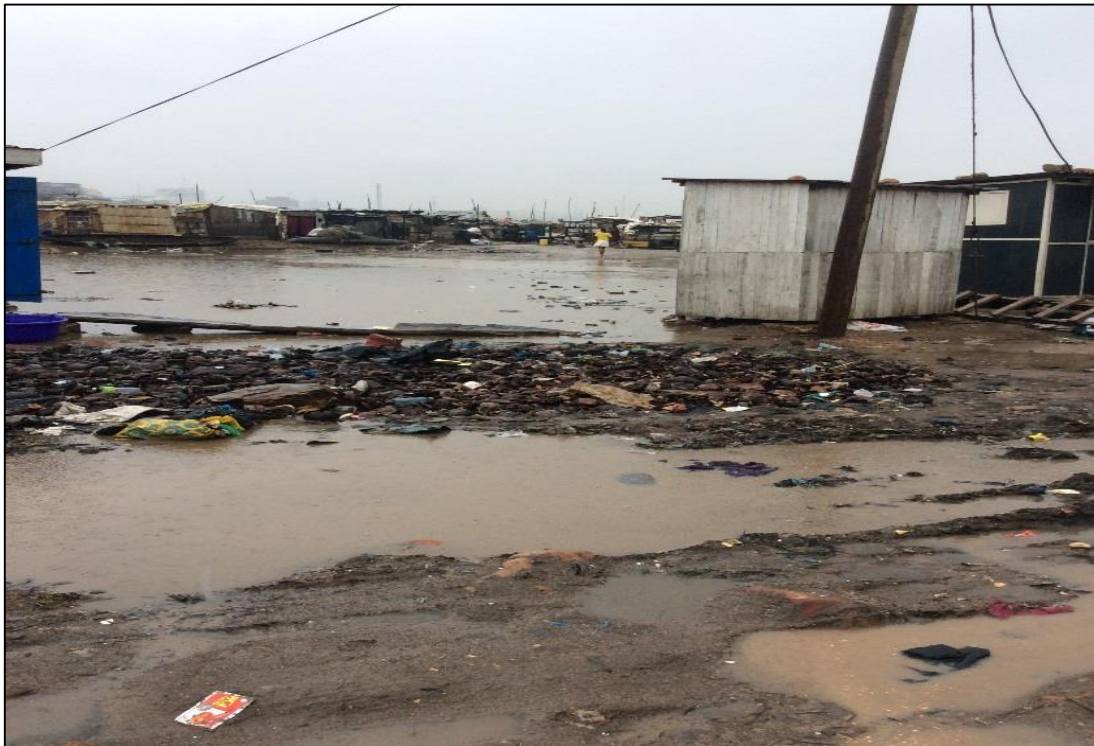
Plate 5.5 Flooding After Normal Rain in Ga-Nshonaa
