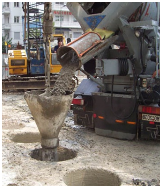
Figure 2.2 Cast-in-place concrete piles (Gary Puntman 2018)
