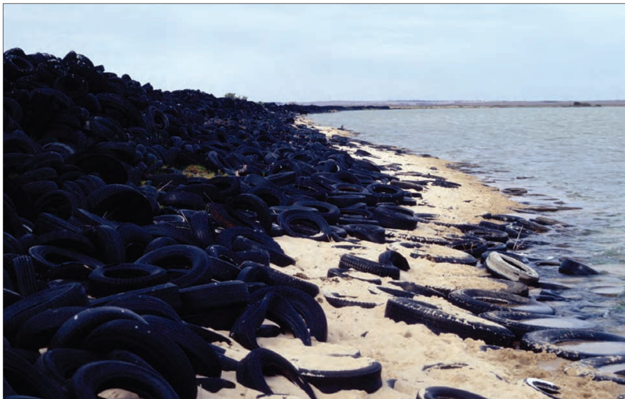
Figure 2.2.16 A tyre wall protecting the sand barrier on the western extremity of the Cooke Plains Embayment. (Photograph by R.P. Bourman)
