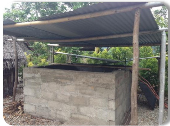
An underground rainwater storage tank (lasitern) built in-situ
