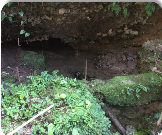
An unprotected spring is the source of water for the Namoru piped water supply
