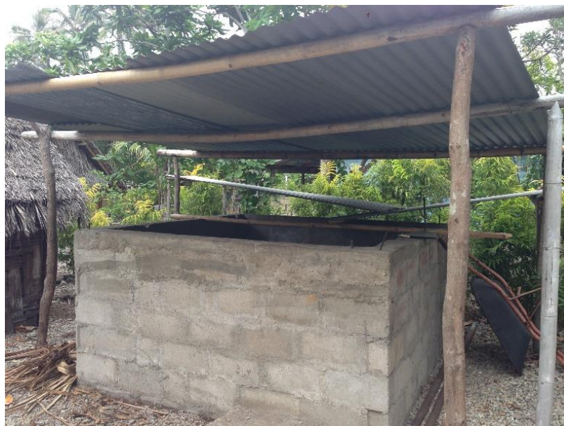
Figure 14. Underground rainwater storage tank (lasitern) in Uripiv
