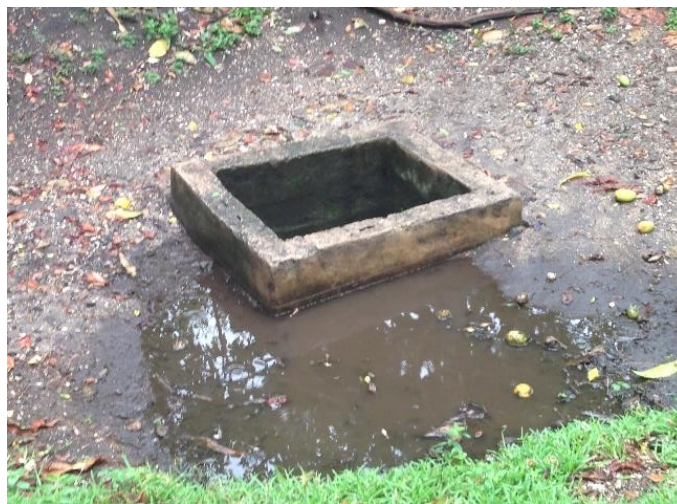
Figure 13. Pooling around well in Uripiv
