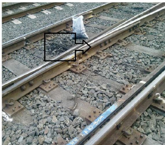
(i) Crossing at Thirroul
