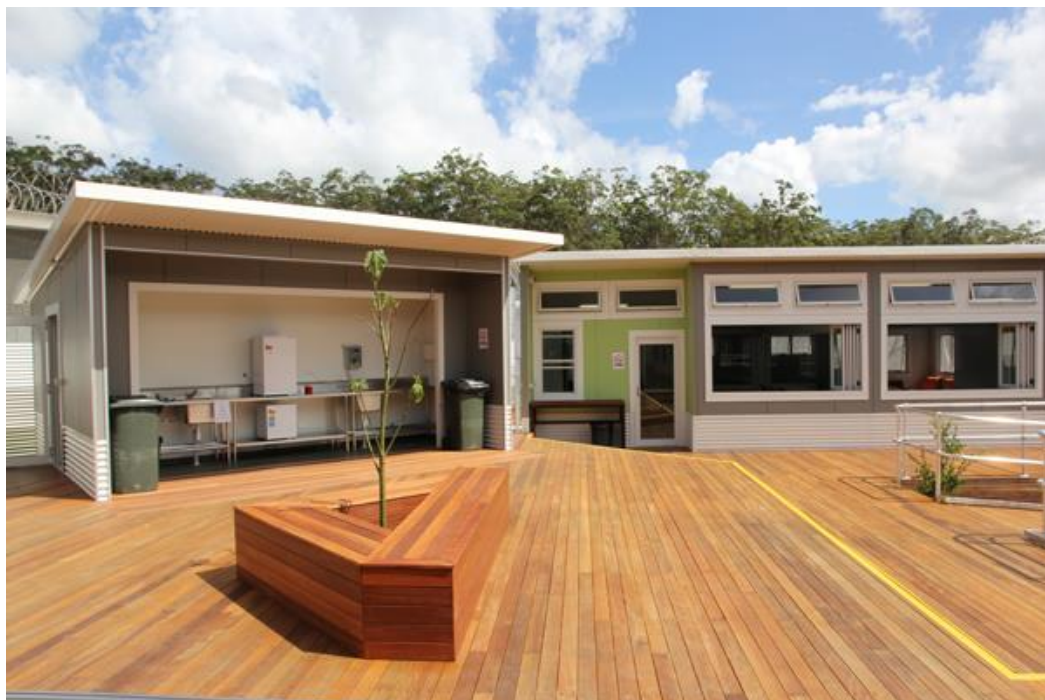
Figure 5 ILC Learner drinks station, open deck and classrooms
