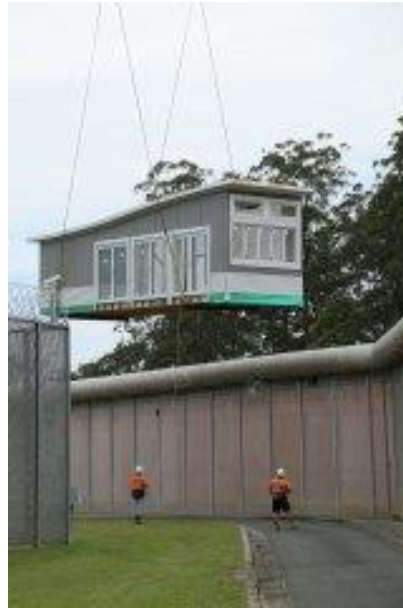
Figure 2 Pre-built ILC module being craned into position 8
