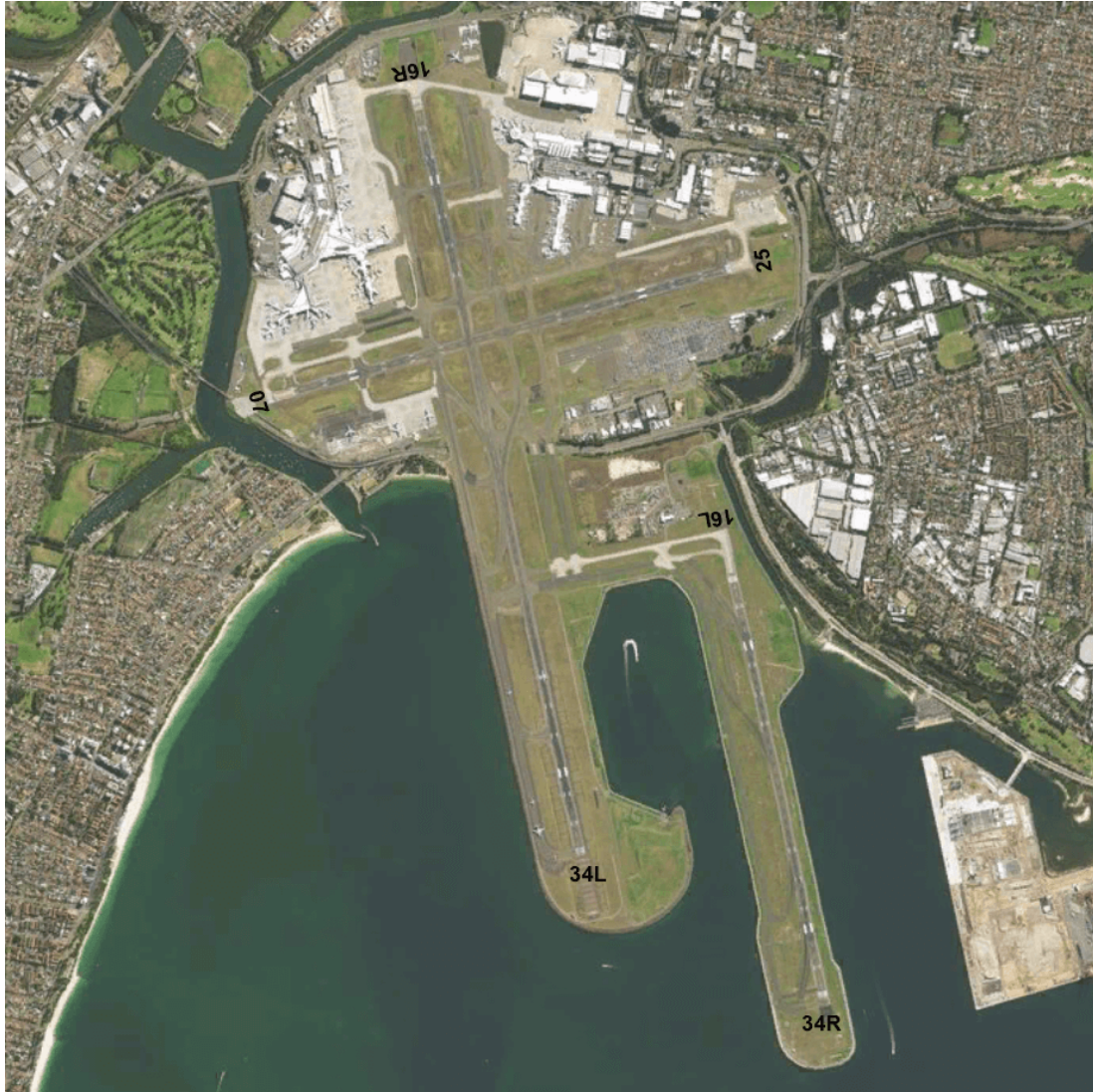
Figure 4: Sydney Airport has three runways: 16R/34L – Main north south runway (3,962m), 16L/34R – Parallel north south runway (2,438m), 07/25 – East west runway (2,530m)
