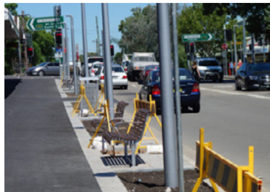
Figure 18: The same street after tree removal. Amenable shade has been lost, seating is in the direct sun and the new paving is slippery when wet. Photo: from the project image bank, collected by the research team during site visits.
