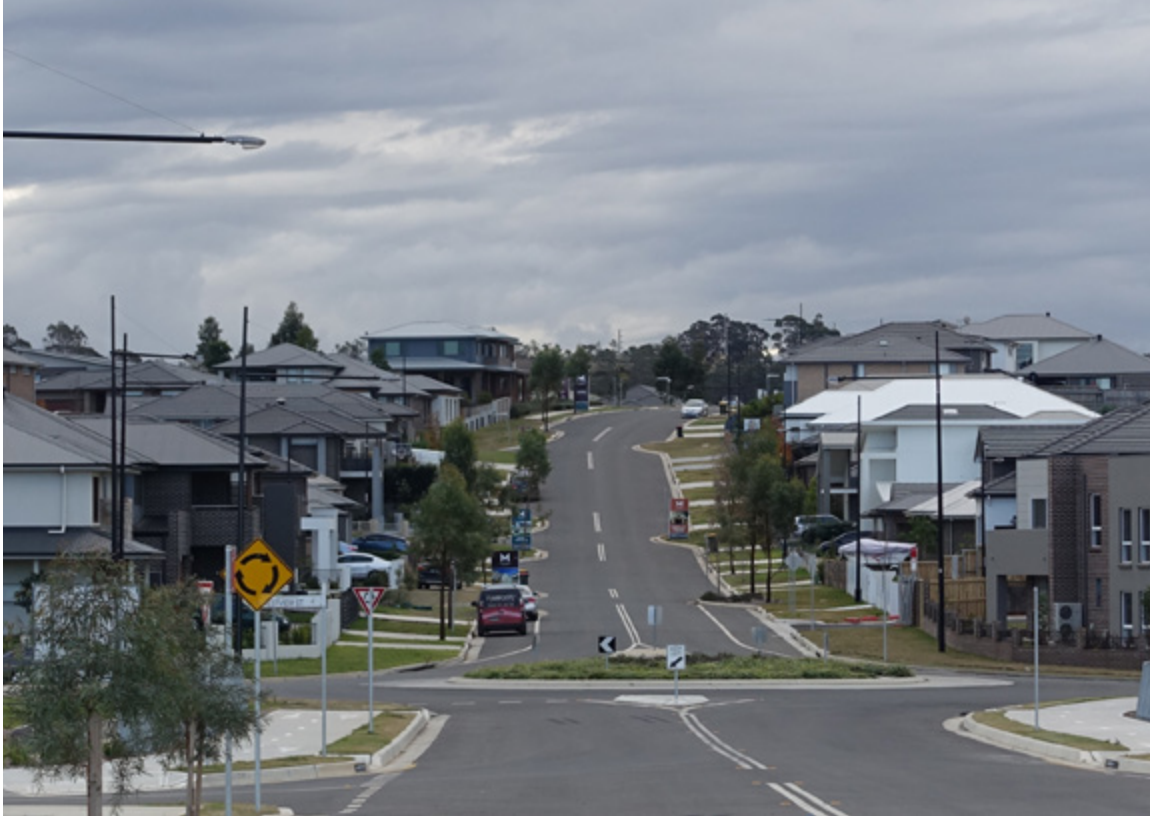
Figure 22: Black top roads and predominance of dark grey roofs absorb heat and increase the demand for air-conditioning in buildings without passive ventilation. Photo: from the project image bank, collected by the research team during site visits.
