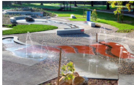
Marrickville water play, Steel Park. A river-side park surrounded by poplar trees. Photo: SDC Engineering http://www.sdcengineering.com.au/marrickville-water-play-park/
