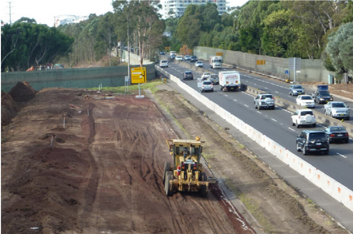
Figure 16: Privileging major roads – clearing the way for M4 widening at Strathfield involved the removal of urban forest planted after the building of the F4 in the early 1980s. Photo: Cathy Jones. Reproduced with permission. https://strathfieldheritage.org/2017/01/31/m4-motorway-history/
