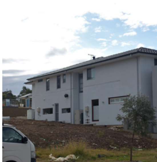
Figure 28: Building to the edge of lot, minimal setbacks, no space for shade trees. Photo: from the project image bank, collected by the research team during site visits.
