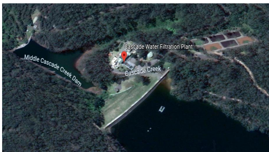
Figure 11. Aerial view of Cascade Water Filtration Plant (google earth, 22/05/2019)
